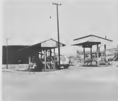
Lego's tank truck loading facilities formerly located east of Lego Heights Gate No. 8, lacked sufficient space needed for safe maneuvering of tank trucks.
